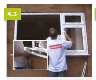
Carefully position the new frame into the aperture. Centralise it and insert packers underneath to level it and maintain the 5mm expansion gap.
