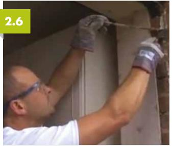
After the removal of the frame, remove all sealant and debris from the brickwork.
