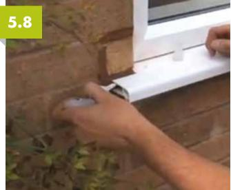
Apply the end cap to the cill using a suitable adhesive.
