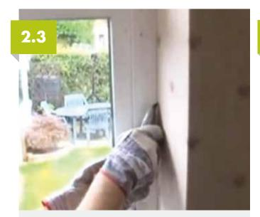
Run a sharp blade around the inside perimeter of the window to break the bond between frame and the plaster. This will also minimise the damage to any interior decoration.
