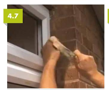
Using a chisel, break off the excess ends of the packers to create a neat finish.
