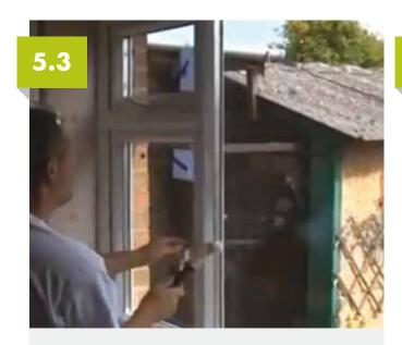
As each pane is positioned, the beading can be installed using a nylon mallet and tapped securely into place. It is recommended that horizontal beads are installed first and that the beads are refitted to their original position.
