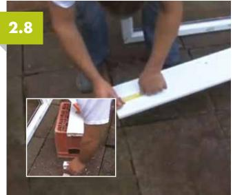
Prepare the external cill for fitting to the new frame. This can be done one of two ways, either fitted full width or rebated around the brickwork to achieve a neat finish.
