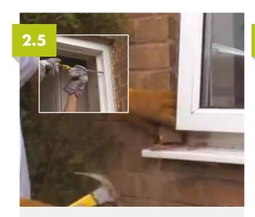
Remove any old fixings and break the external silicone seal with a blade. Also remove the external brick corners to release the old frame.
