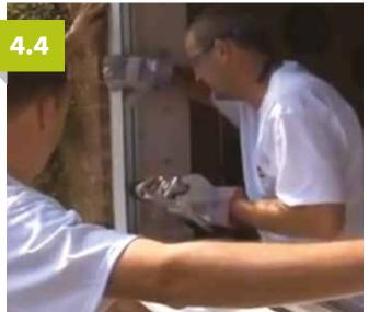
Check that frame is both level and plumb, then drill fixing holes into the frame sides. These should be drilled approximately 150mm from the top and bottom corners and approximately 600mm in between (a minimum of 2 fixings per side)
