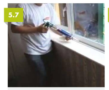
Ensure that any trims are bonded to the frames to prevent dirt entering the joint.
