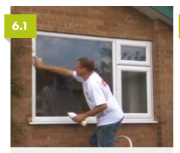
Clean the external surfaces to remove the dirt and grit.
